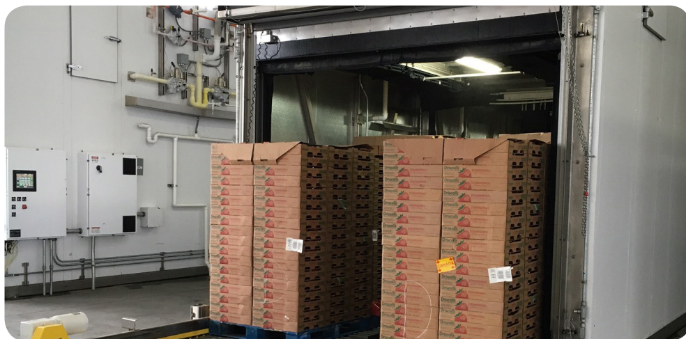
The Modular Automated Cooling System at D'Arrigo Bros. only takes about two hours to cool eight pallets worth of product.
